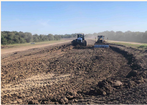
Raising a levee with new fill.
